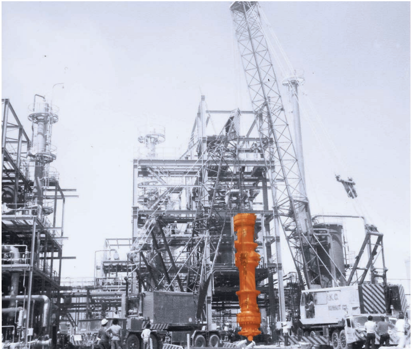
Late seventies, Kuwait Melamine plant under construction
