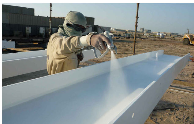
Figure 3. Example of intumescent fire protection system used to seal penetrations and protect structures.
